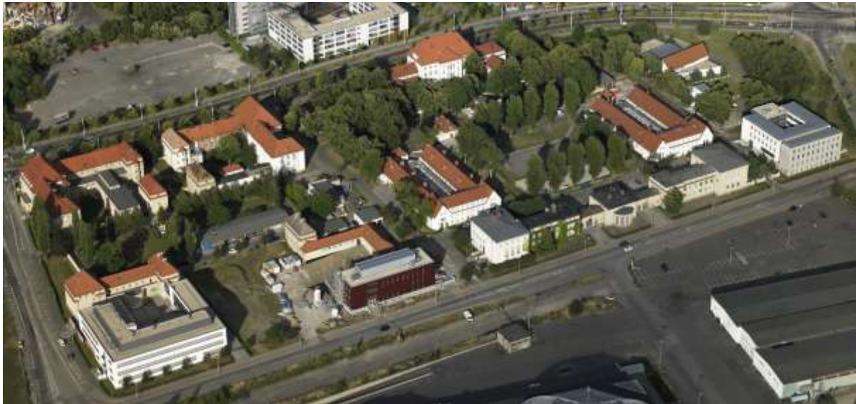
Aerial view of VMF
